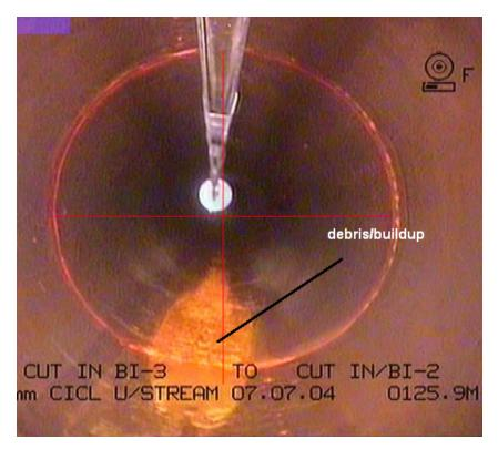
At 126m, there is some debris in the pipe, causing the diameter to reduce to 1115mm. However, the diameter increases to a more realistic minimum of 1131mm at 129m (131.25) from BI-3.
